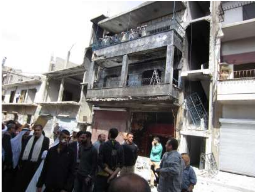
Buildings in Homs Destroyed by car bomb.
